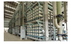
Always follow the membrane manufacturer's recommendations for pH, cleaning temperature and contact time.
